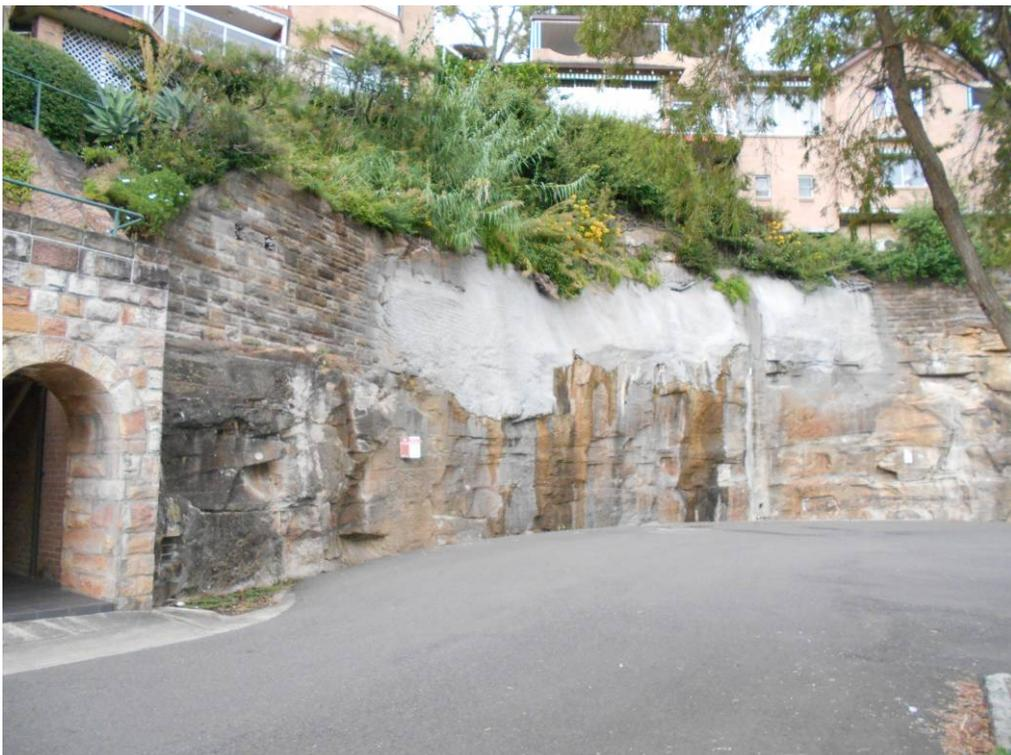
**Figure 4.3** South-east facing view of the escarpment wall. Note the garage entrance on the eastern (left) part of the escarpment wall, and the construction of retaining walls and the use of concrete on the remainder of the escarpment wall.
